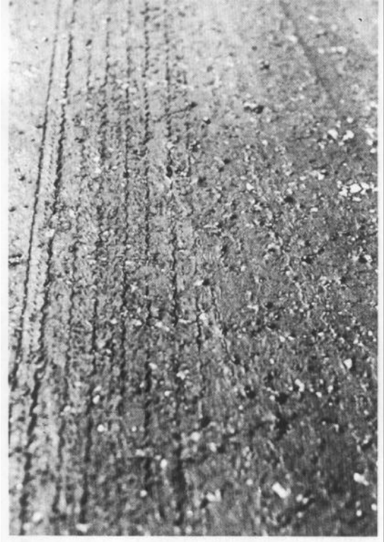
Figure 11. High-severity bleeding
