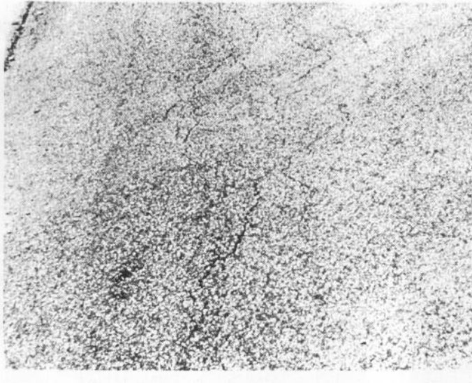
Figure 2. Low-severity alligator cracking
