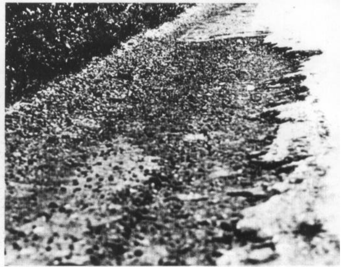
Figure 31. High-severity edge cracking
