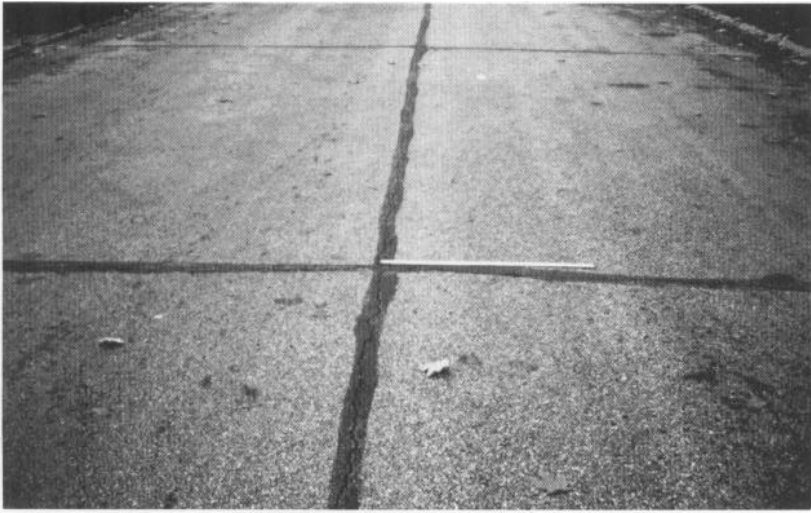
Figure 32. Low-severity joint reflection cracking
