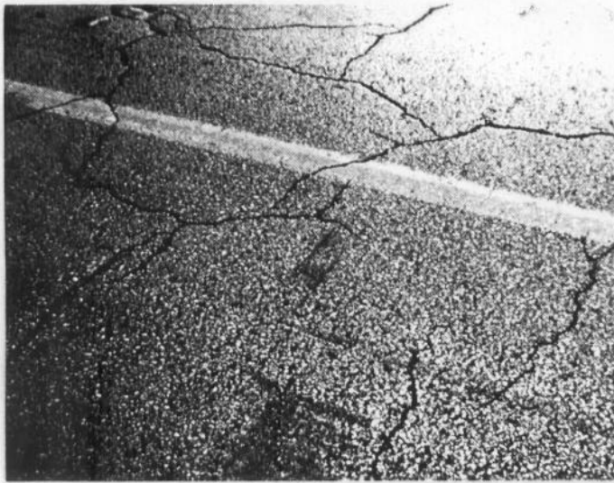
Figure 14. Medium-severity block cracking
