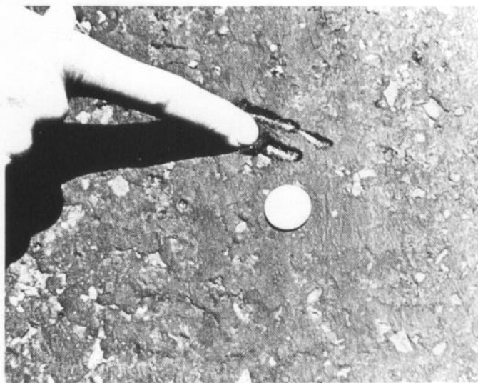
Figure 10. Medium-severity bleeding
