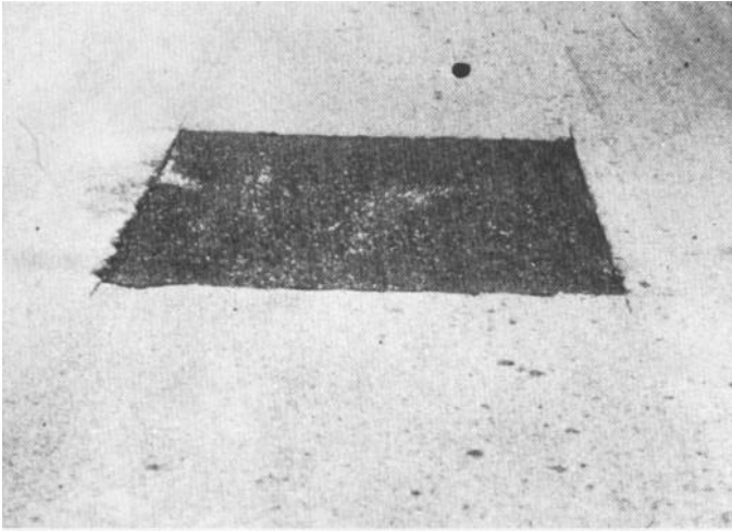
Figure 43. Low-severity patching and utility cut patching
