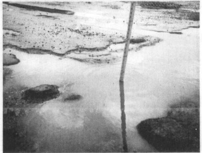
Figure 52. High-severity pothole
