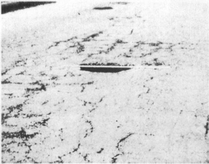
Figure 51. Medium-severity pothole
