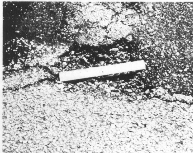
Figure 50. Low-severity pothole
