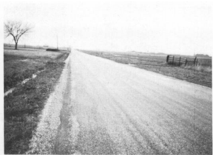
Figure 21. Low-severity corrugation
