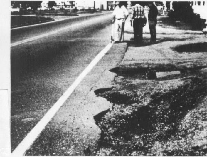
Figure 30. High-severity edge cracking
