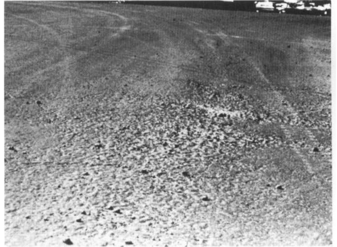
Figure 71. Medium-severity weathering and raveling
