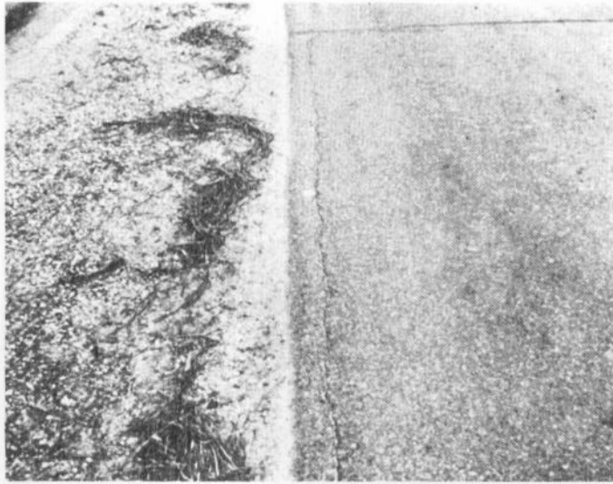
Figure 28. Low-severity edge cracking
