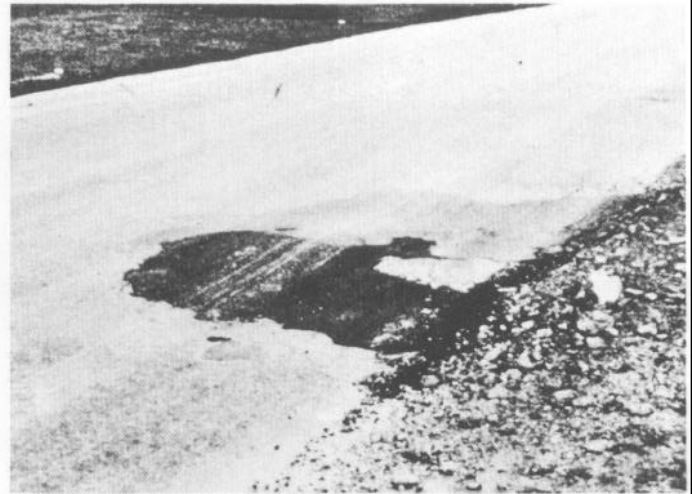
Figure 46. Medium-severity patch
