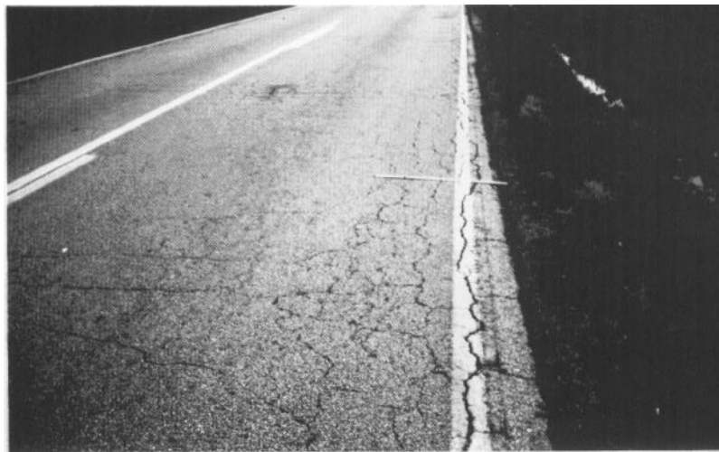
Figure 5. Medium-severity alligator cracking
