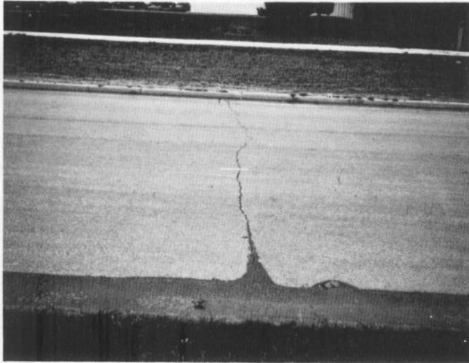
Figure 39. Low-severity longitudinal and transverse cracking
