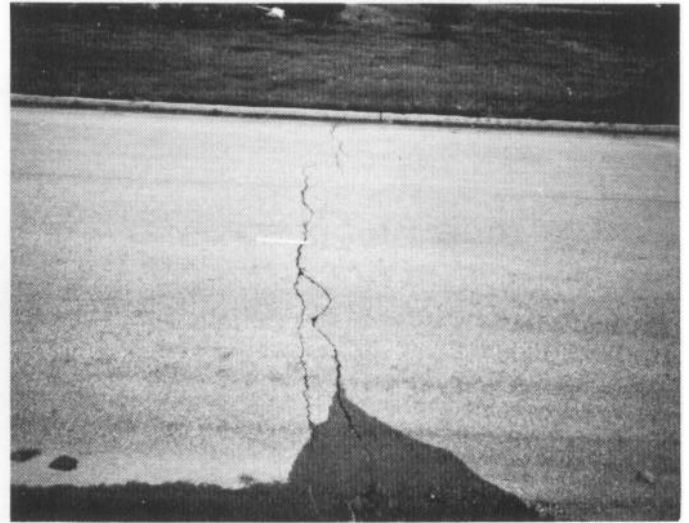
Figure 40. Medium-severity longitudinal and transverse cracking
