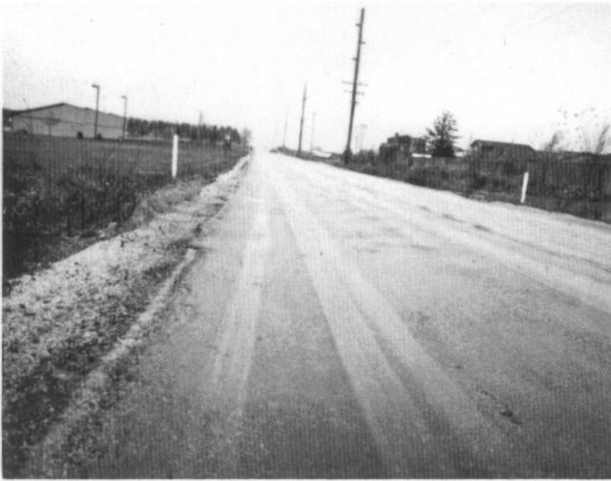
Figure 23. Medium-severity corrugation
