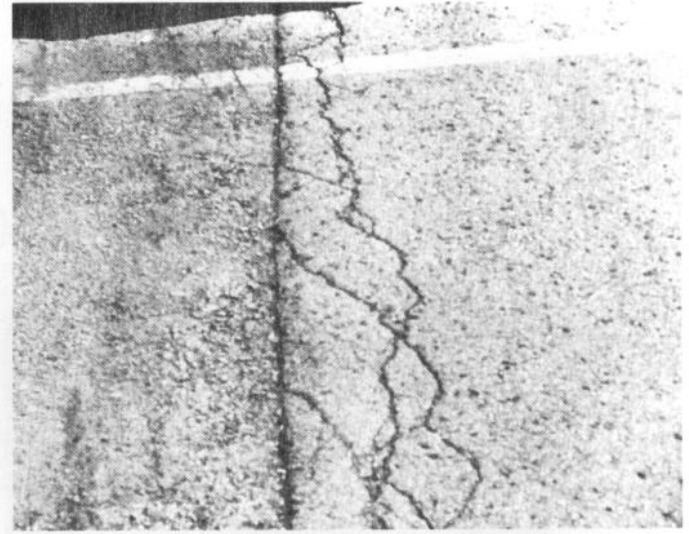
Figure 29. Medium-severity edge cracking
