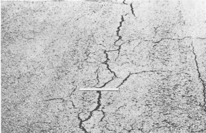
Figure 41. Medium-severity longitudinal and transverse cracking [ \frac{3}{4} in (19 mm) crack surrounded by light random cracks].
