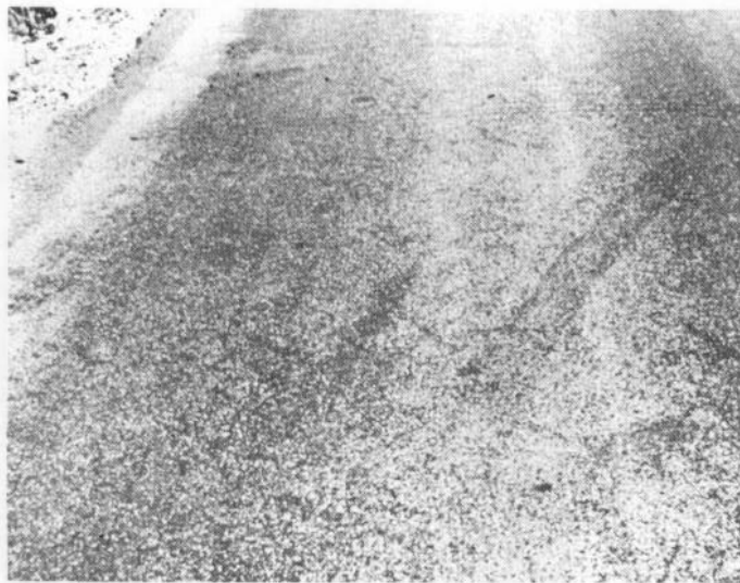
Figure 9. Low-severity bleeding
