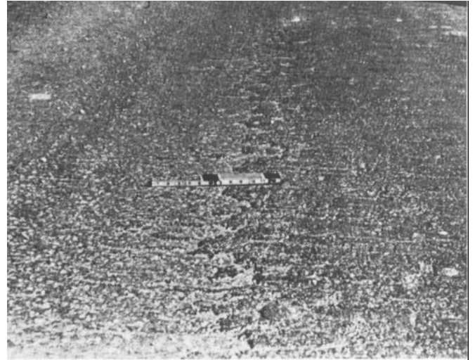
Figure 69. Low-severity weathering and raveling caused by tracked vehicles
