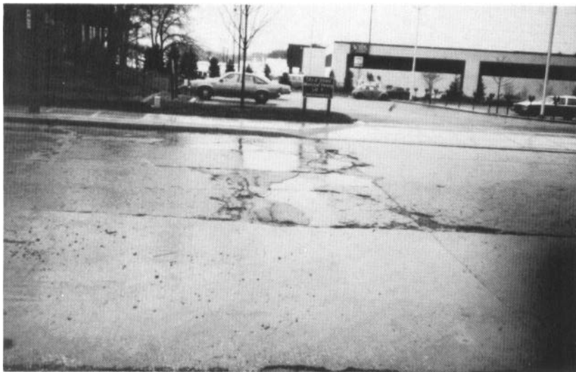
Figure 47. High-severity patching and utility cut patching
