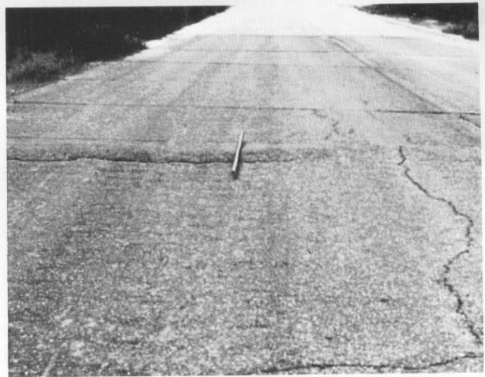
Figure 19. Medium-severity bumps and sags
