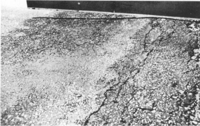
Figure 20. High-severity bumps and sags
