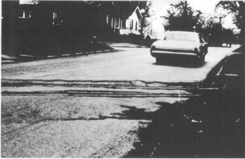
Figure 56. High-severity railroad crossing
