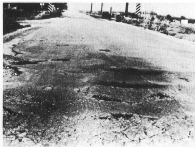
Figure 62. Medium-severity shoving approaching high severity
