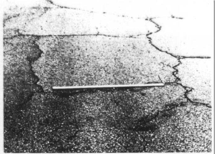
Figure 13. Medium-severity block cracking
