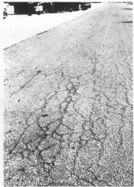
Figure 4. Medium-severity alligator cracking
