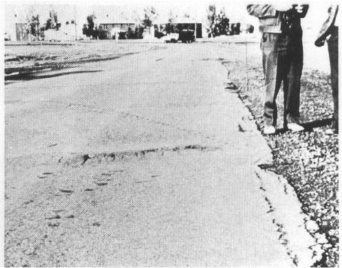
Figure 17. Medium-severity bumps and sags
