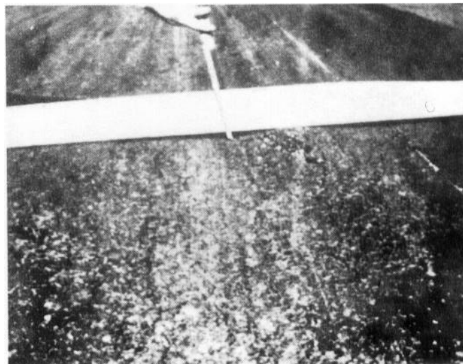
Figure 70. High severity rutting (note alligator cracking associated with rutting)
