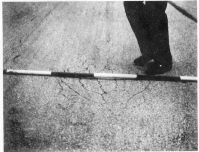
Figure 5. Medium severity alligator cracking, (note the depression occurring with the cracking)
