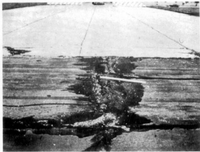
Figure 79. High severity swell
