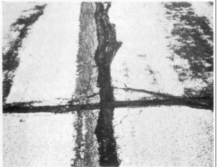
Figure 36. Medium severity joint reflection cracking
