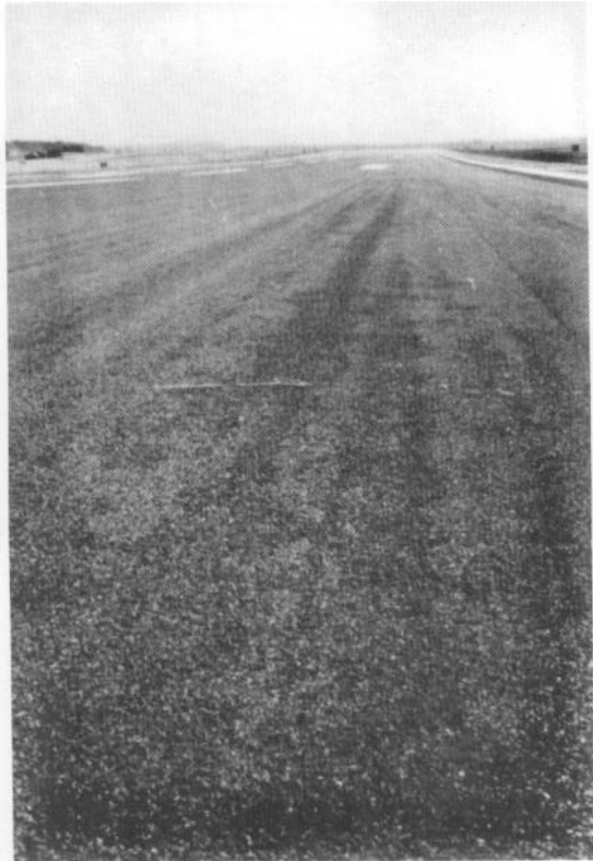
Figure 65. Medium severity raveling/ weathering showing rough and pitted surface
