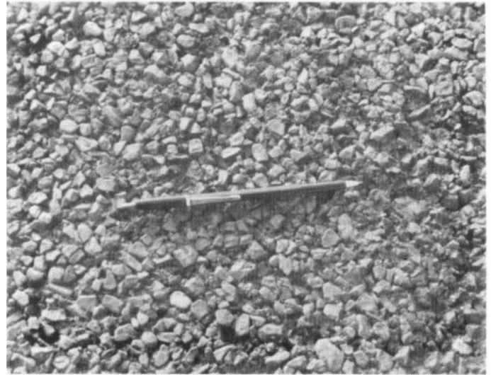
Figure 64. Medium severity raveling/weathering on a porous friction course surface
