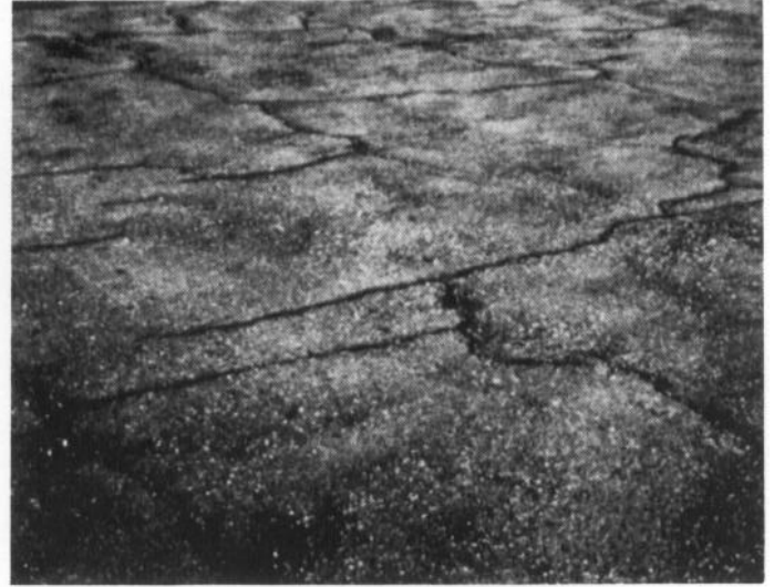
Figure 18. Medium severity block cracking
