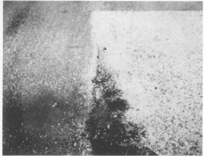
Figure 52. Medium severity patch
