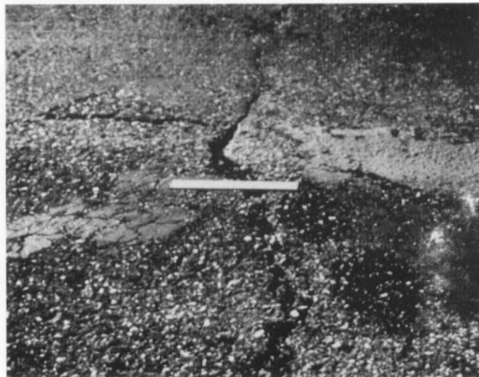
Figure 43. High severity longitudinal crack
