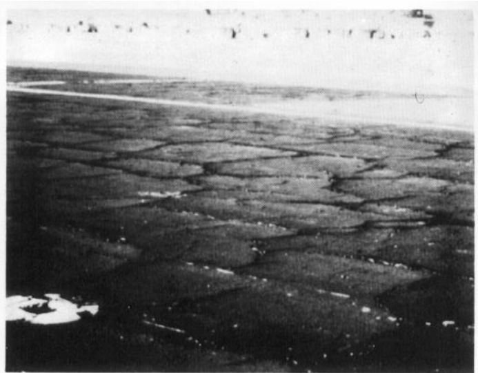
Figure 20. High severity block cracking
