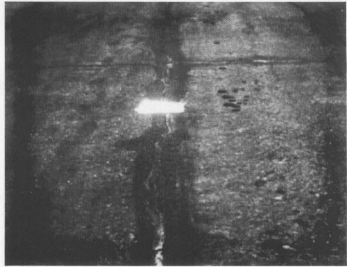
Figure 41. Medium severity longitudinal crack, (note the crack is reflective but not at the joint of slab)
