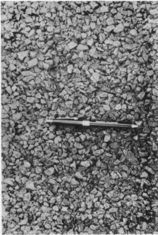
Figure 61. Typical porous friction course surface with no raveling/weathering
