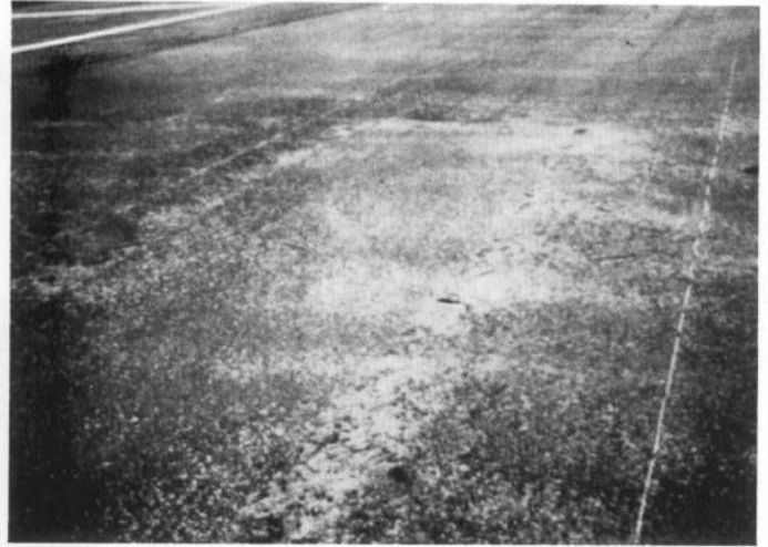
Figure 23. Medium severity corrugation
