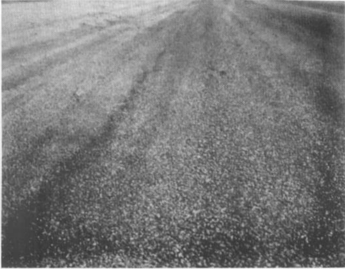
Figure 55. Low severity raveling/weathering
