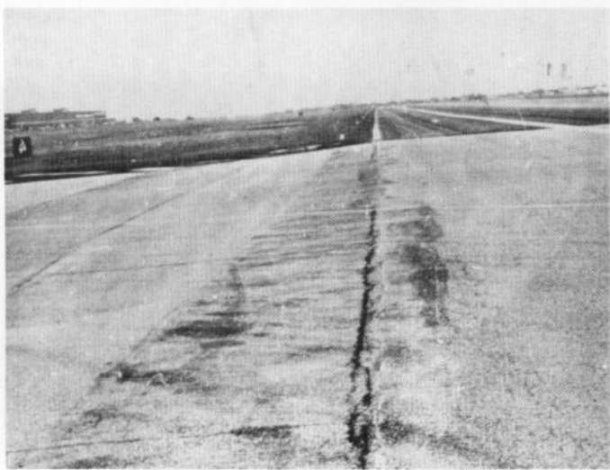
Figure 72. This photograph shows a shove of low severity on the outside and medium severity in the middle
