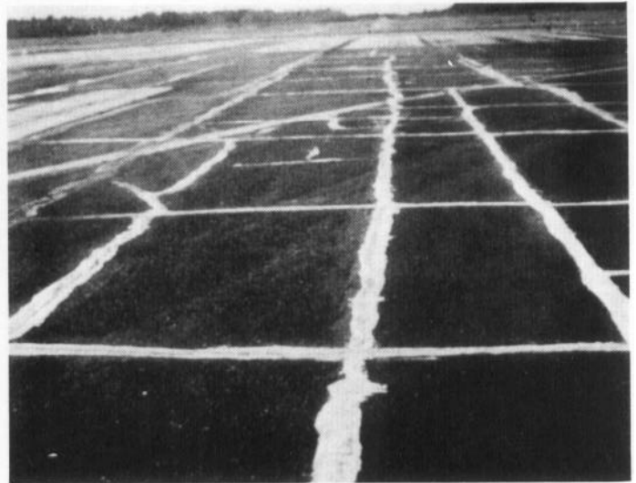
Figure 14. Low severity block cracking, filled cracks
