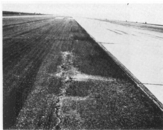
Figure 42. Medium severity longitudinal crack
