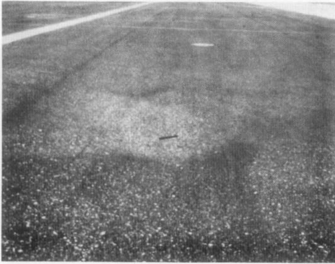
Figure 27. Medium severity depression
