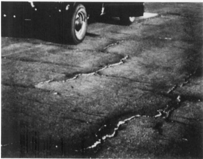
Figure 19. High severity block cracking
