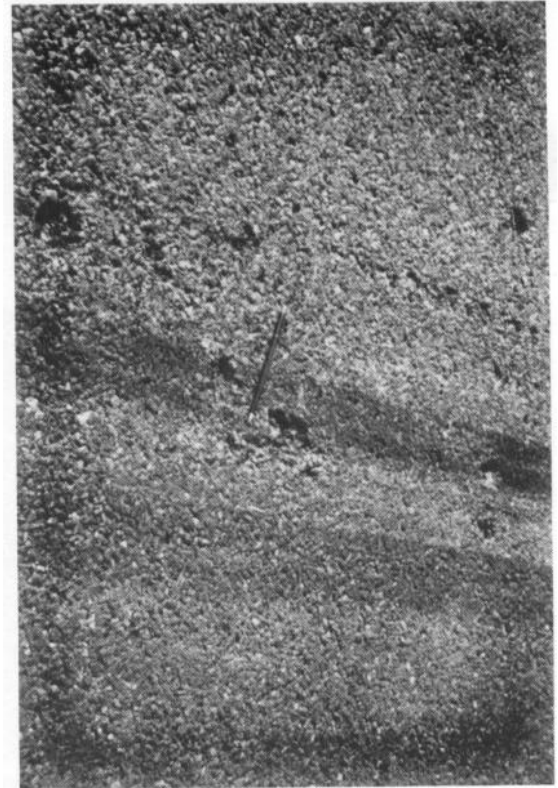
Figure 66. High severity raveling/weathering on a porous friction course surface
