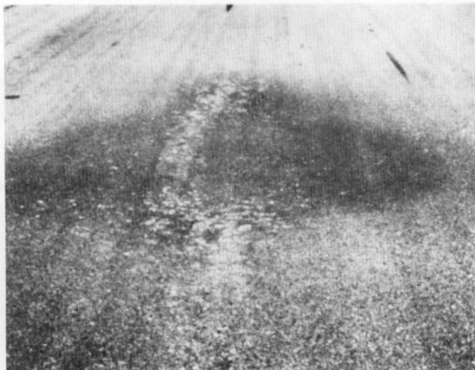
Figure 25. Low severity depression
