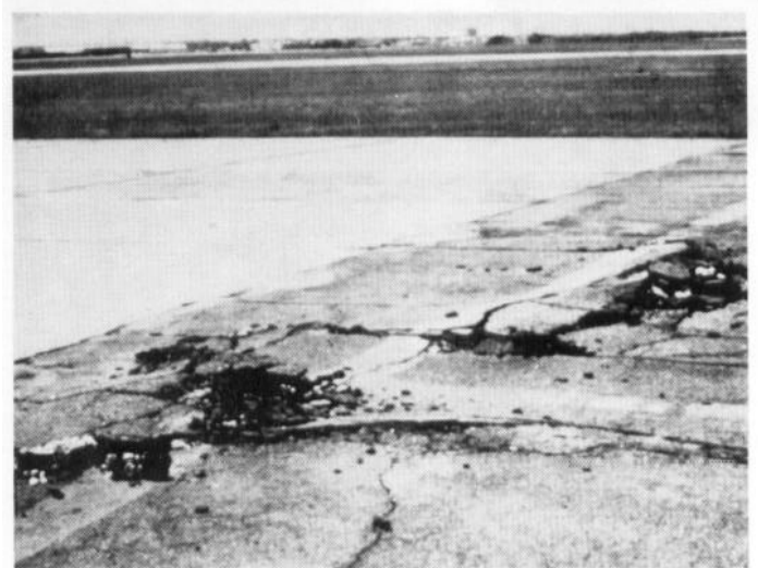
Figure 73. High severity shoving
