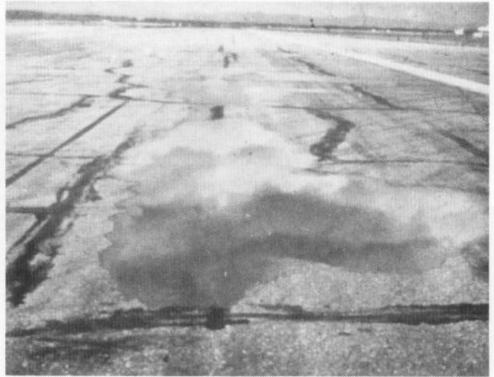
Figure 28. High severity depression (2 inches)
