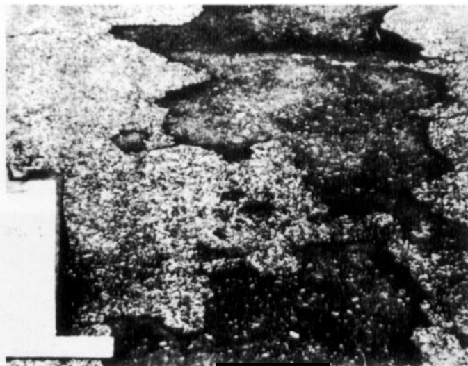
Figure 60. High severity raveling/weathering
