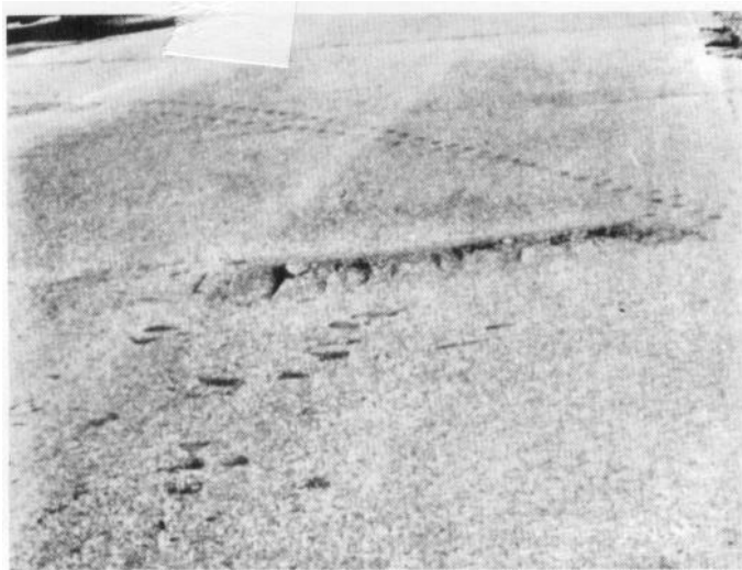
Figure 78. High severity swell
