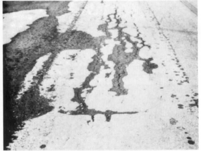
Figure 3. Low severity alligator cracking
