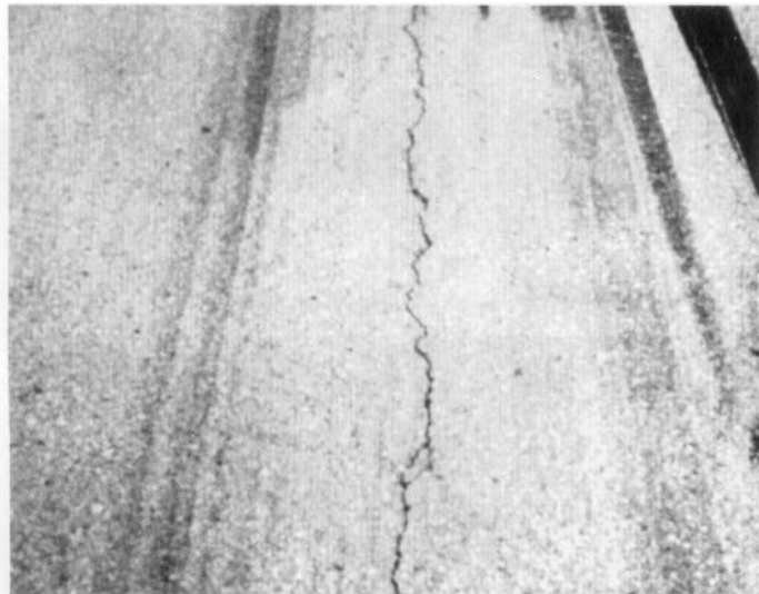
Figure 33. Low severity joint reflection cracking, nonfilled crack
