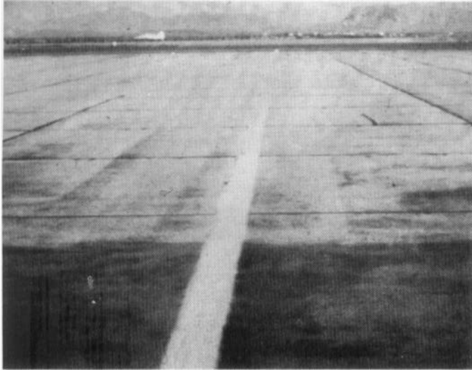
Figure 31. Low severity joint reflection cracking
