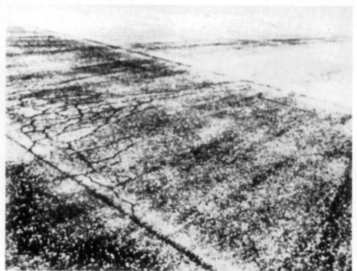
Figure 9. Medium severity alligator cracking, approaching high severity
