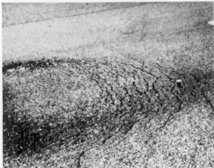
Figure 74. Slippage cracking
