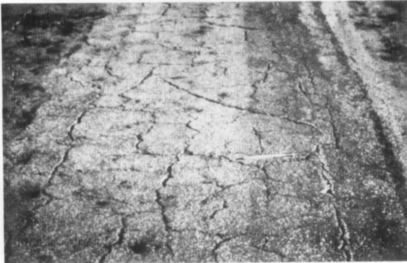
Figure 21. High severity block cracking
